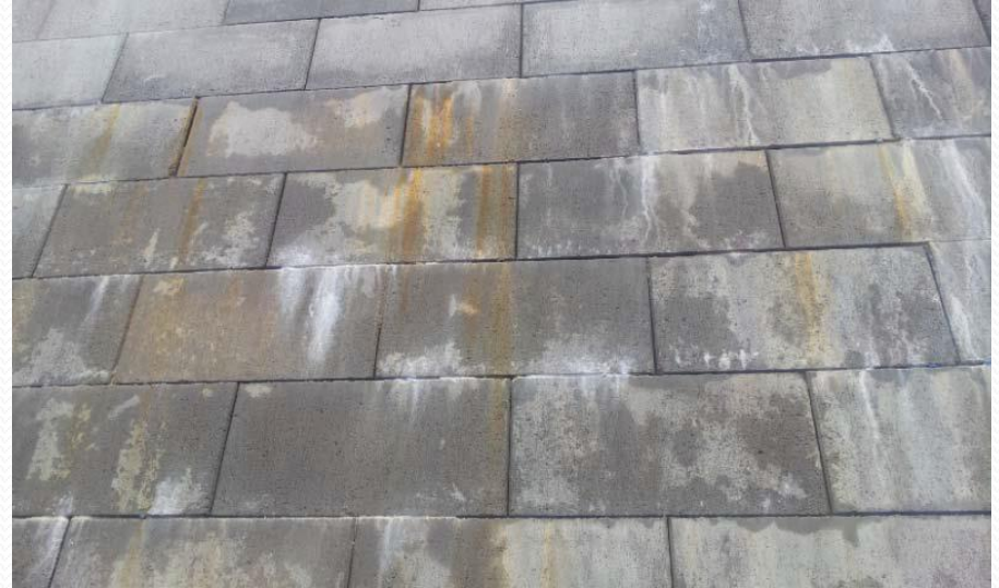
Dampness of wall, rust and efflorescence
