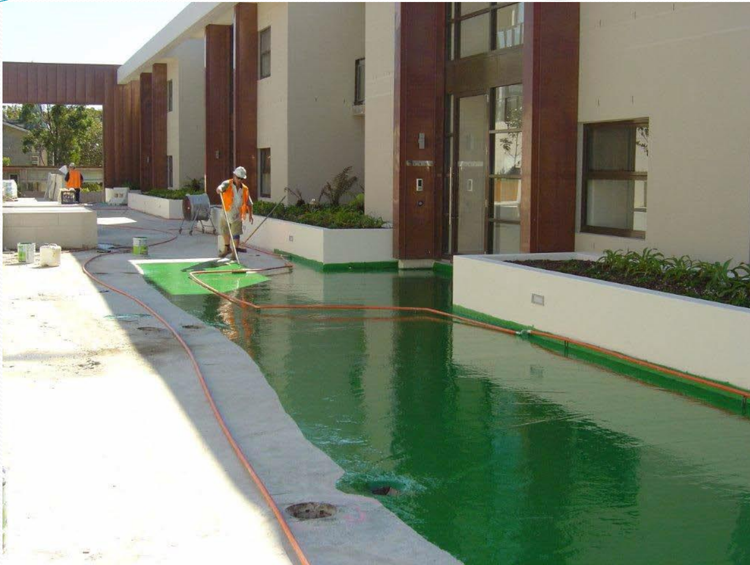
Liquid Membrane – Applied on a podium by Rollers
