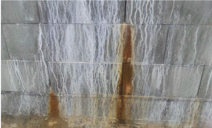
Leaching of efflorescence and signs of rust
