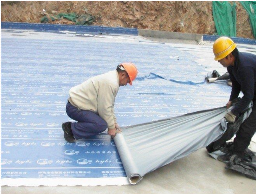
Self-adhesive waterproofing Sheet membrane
