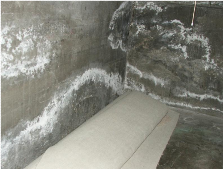
Efflorescence
