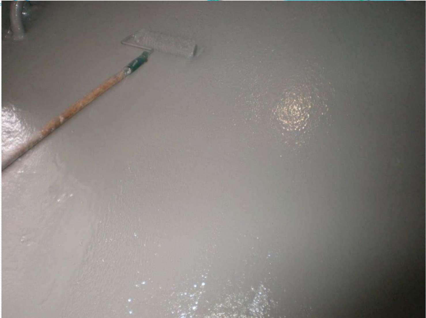
Liquid Membrane – Applied by Rollers
