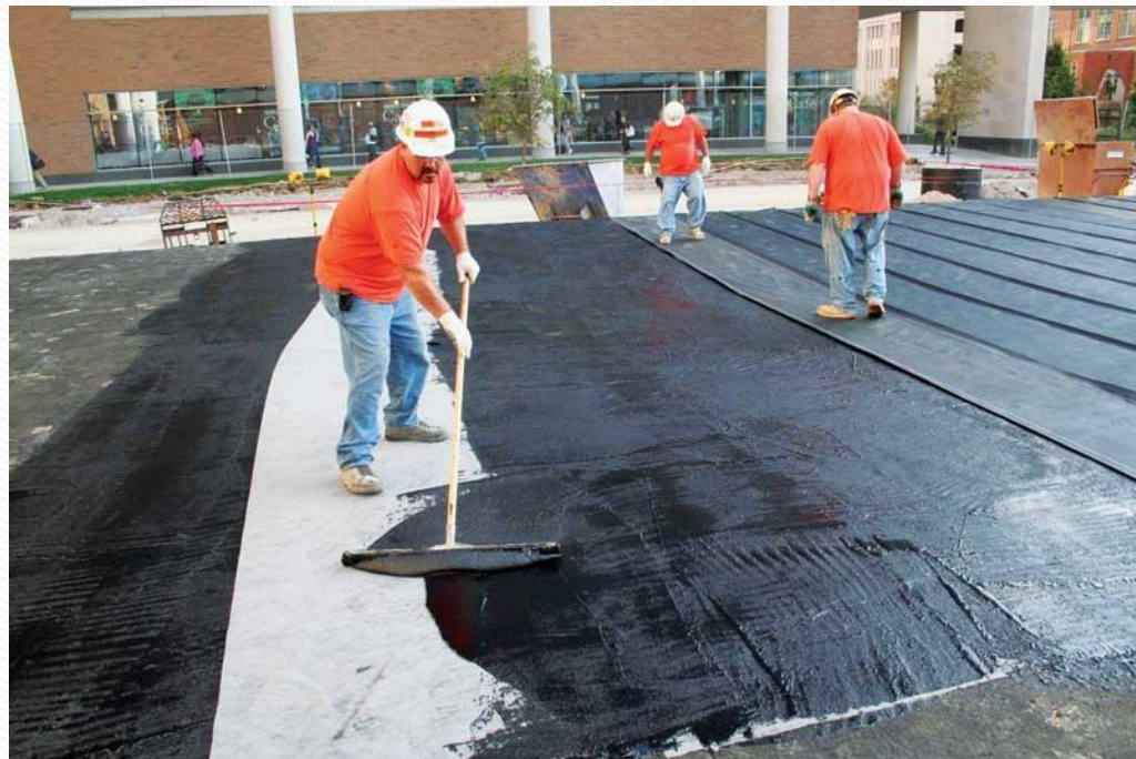
Hot-applied rubberized bitumen
