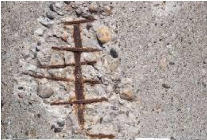
Reinforcement Corrosion
